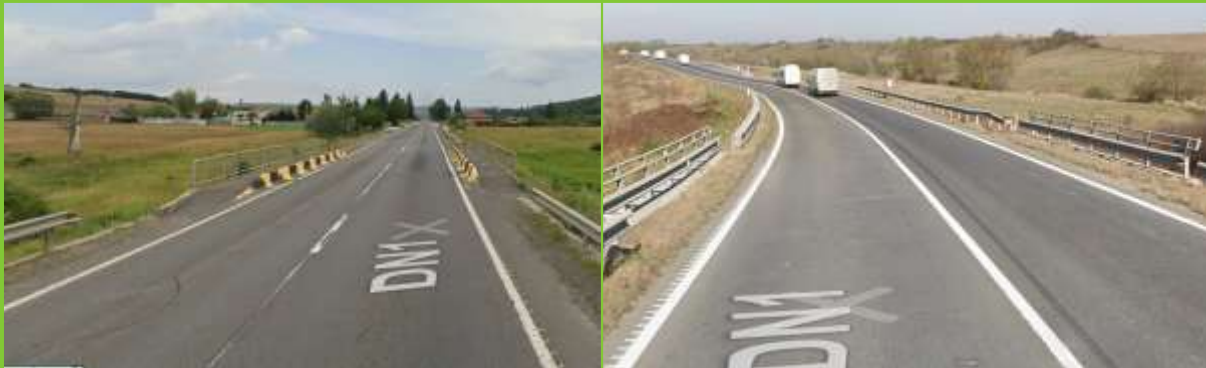
Examples of hazardous safety barriers ends
