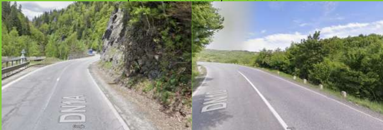
Examples of hazardous safety barriers ends
