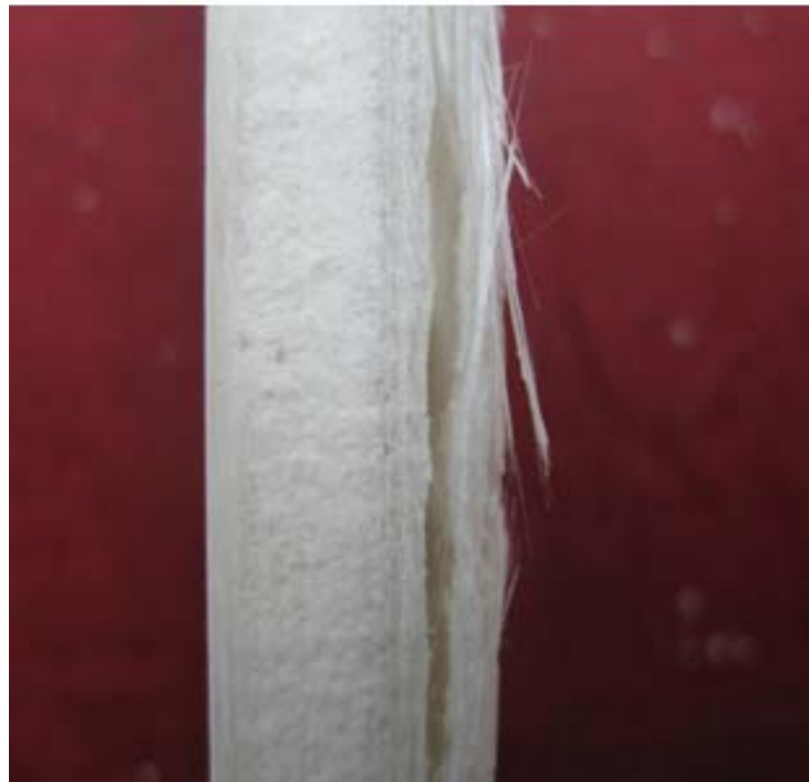
Figure 3.43. Typical failure mode in side view 1
